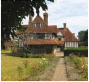
Timber Framed House
