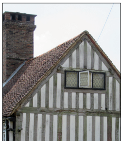
Timber framed buildings
