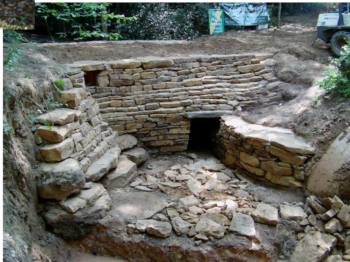
Strawberry Wood Culvert after it was restored
