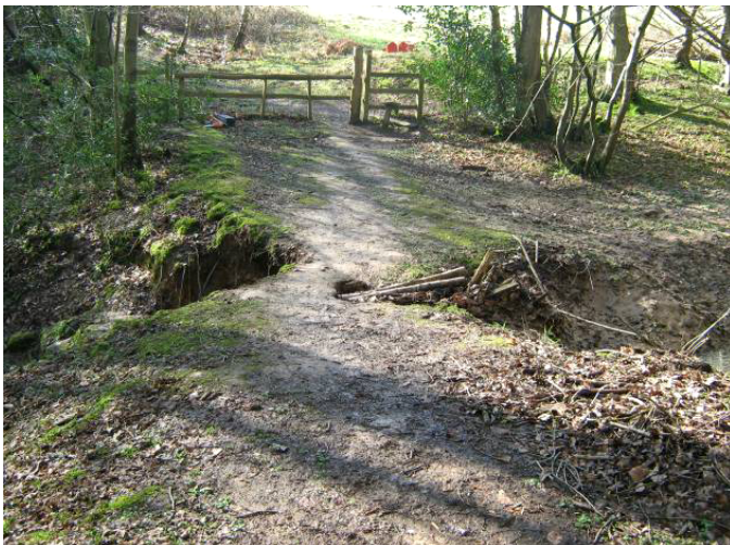
Strawberry Wood Culvert before it was restored
