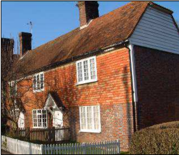
A typical Wealden cottage
