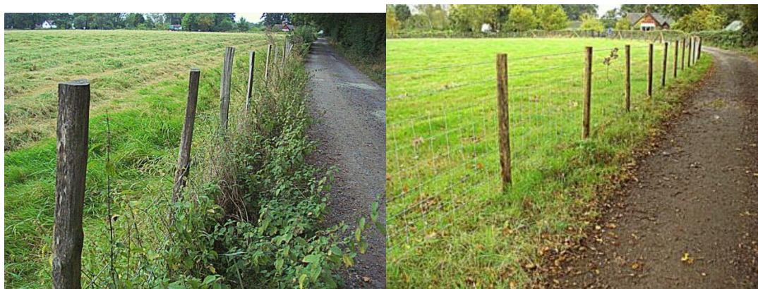
Figure 4: Installing missing infrastructure – before and after fence replacement, near Tonbridge
