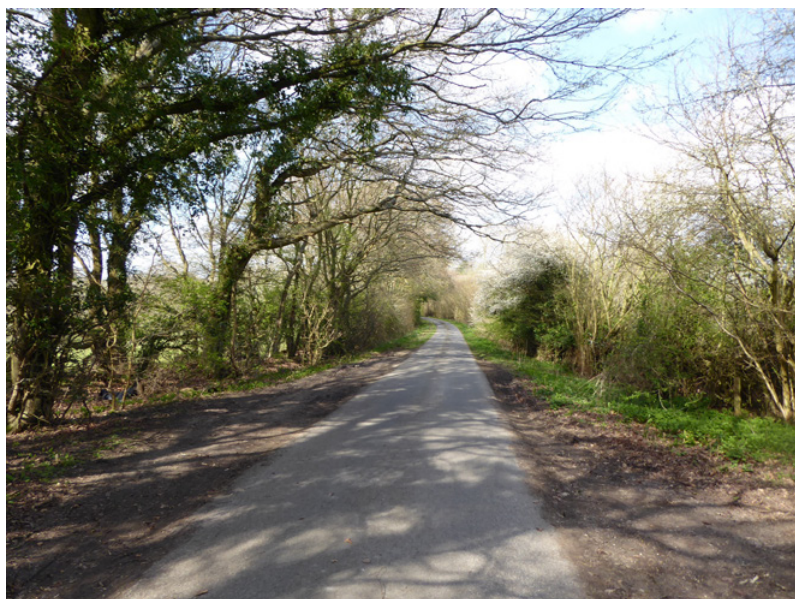
An early 19th century road raised above the surrounding ground level, with ditches for drainage to either side. Photo © J Lake
