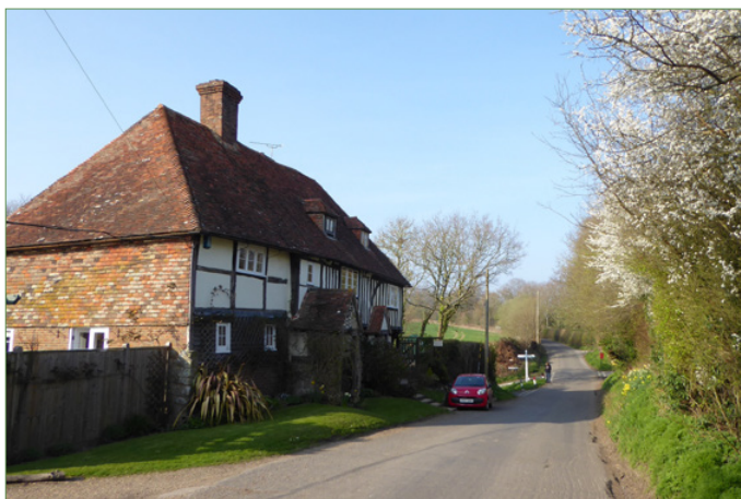
Four Wents (see map on page 38) from the south. This 15th century house is prominently positioned at a road junction, with no expense spared on its close-studded timber frame elevations; the fine front porch was added in 1681. Photo © J Lake
