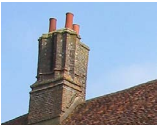
Chimneystacks articulating roofscapes
