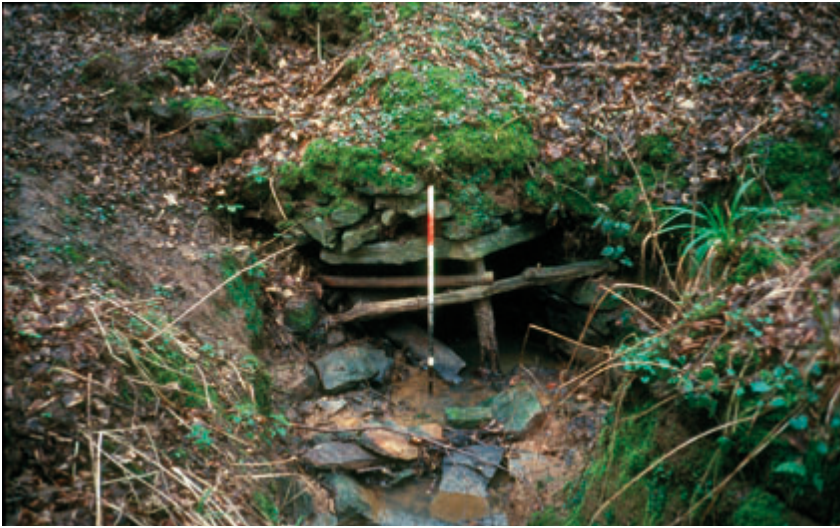
Culvert at Strawberry Wood, near Benenden in the High Weald (photo - NB)
