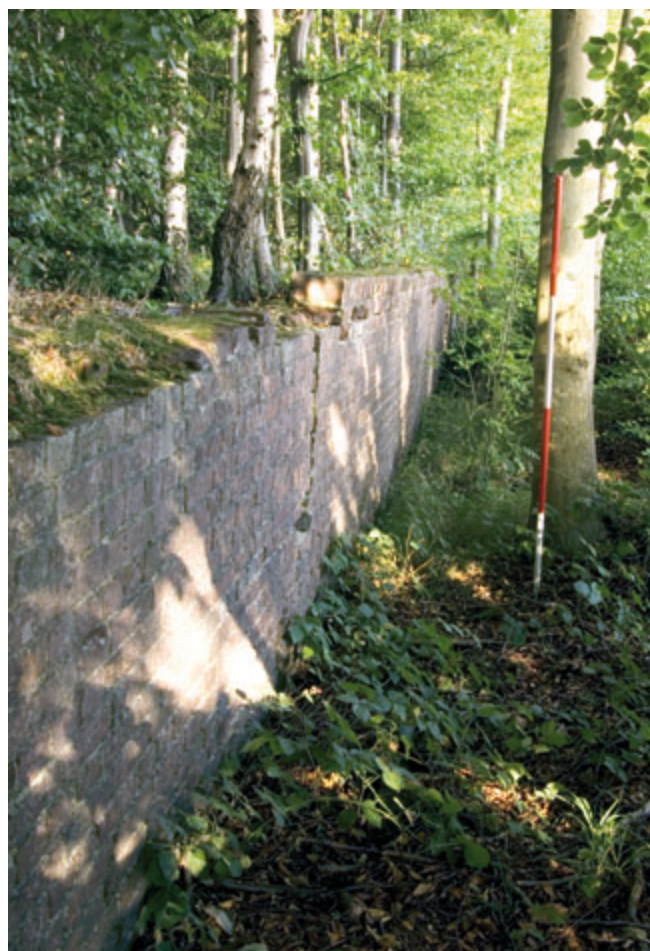
Deer leap at Godmersham Park in the Kent Downs, lying between the park boundary and Kings Wood. The leap is 1.5 metres high, and its ditch, on the park side, is 1.5 metres wide. (photo - PM)
