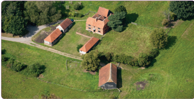
This group in the Low Weald has the house facing into a yard. To the rear of the house is a back kitchen, illustrated on p.33, and in front of the yard is a barn with a lean-to for cattle.(© English Heritage NMR 27205-005)
