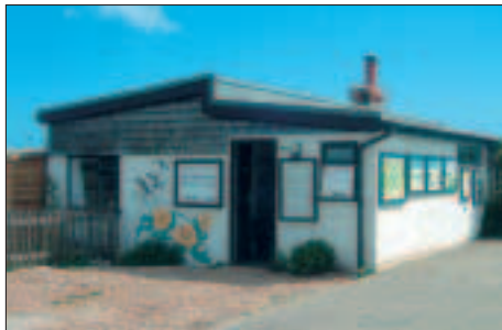
Lime Kiln Cottage Information Centre
