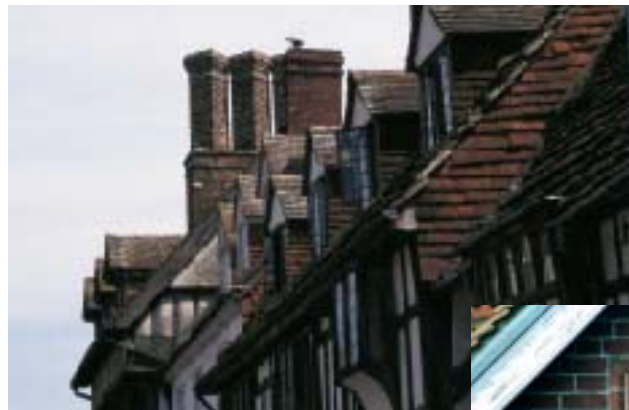
Chimney pots demonstrate the versatility of brick
