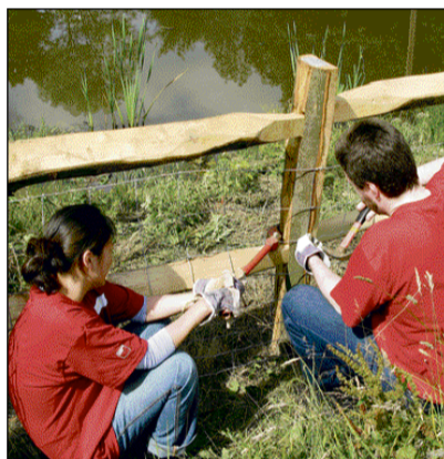
Team work helps with constructing traditional chestnut fencing
