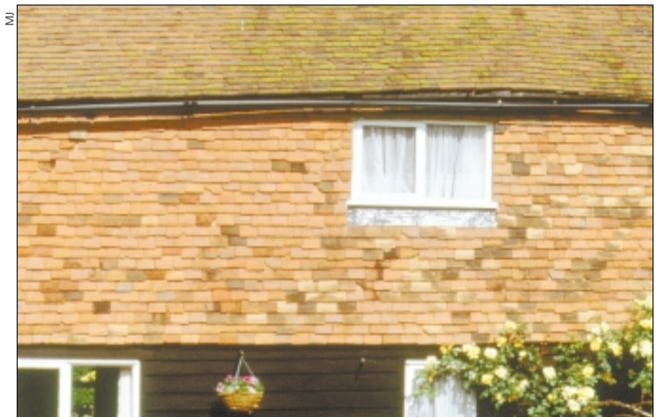
Tile hanging on a timber-framed house
