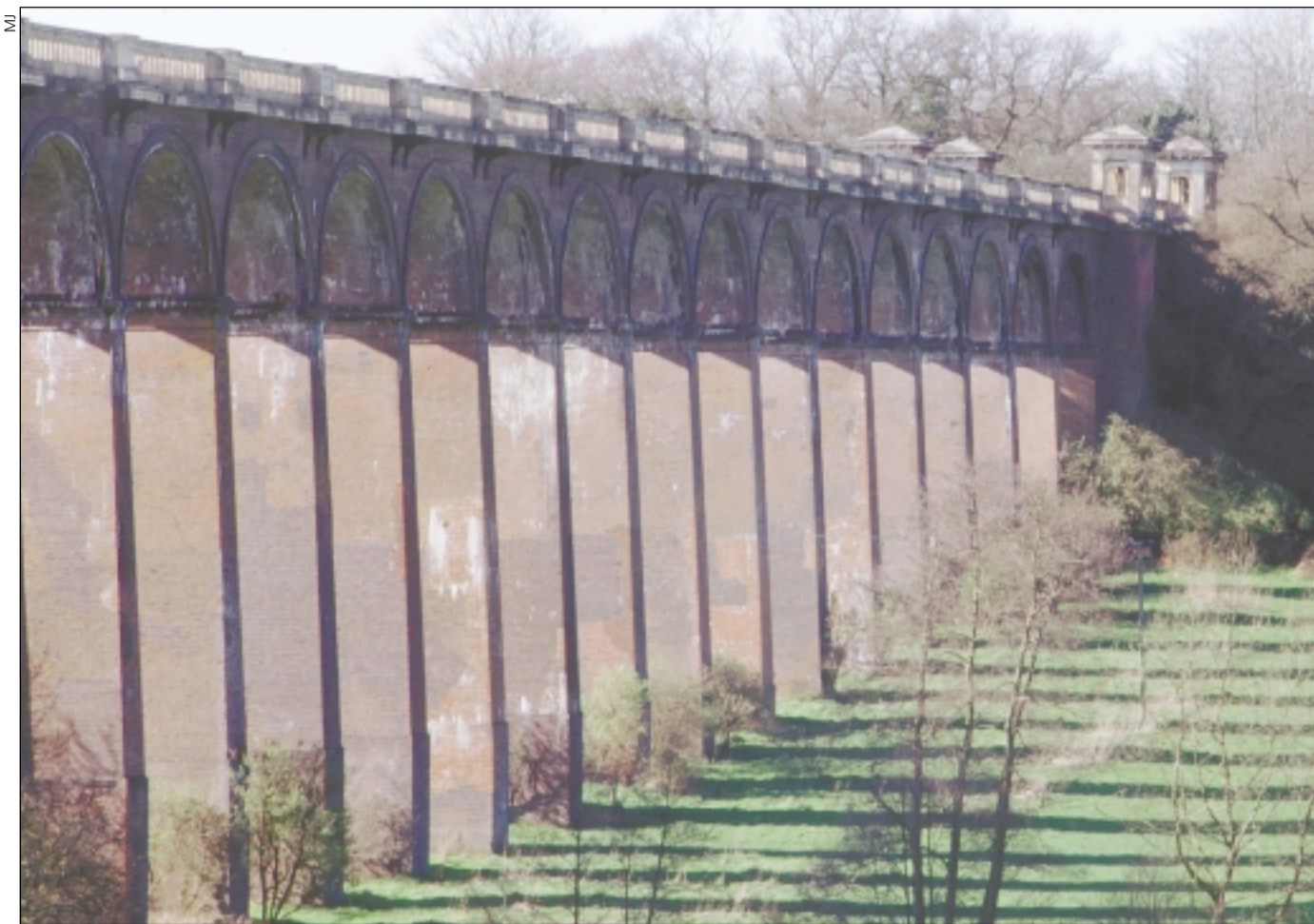
Balcombe Viaduct – built with 11 million bricks
