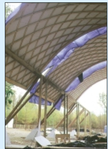
The Woodland Enterprise Centre building (above) is a revolutionary new gridshell building being constructed out of local timbers at Flimwell, East Sussex
