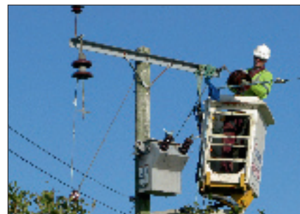
Overhead power line removal at Brightling
