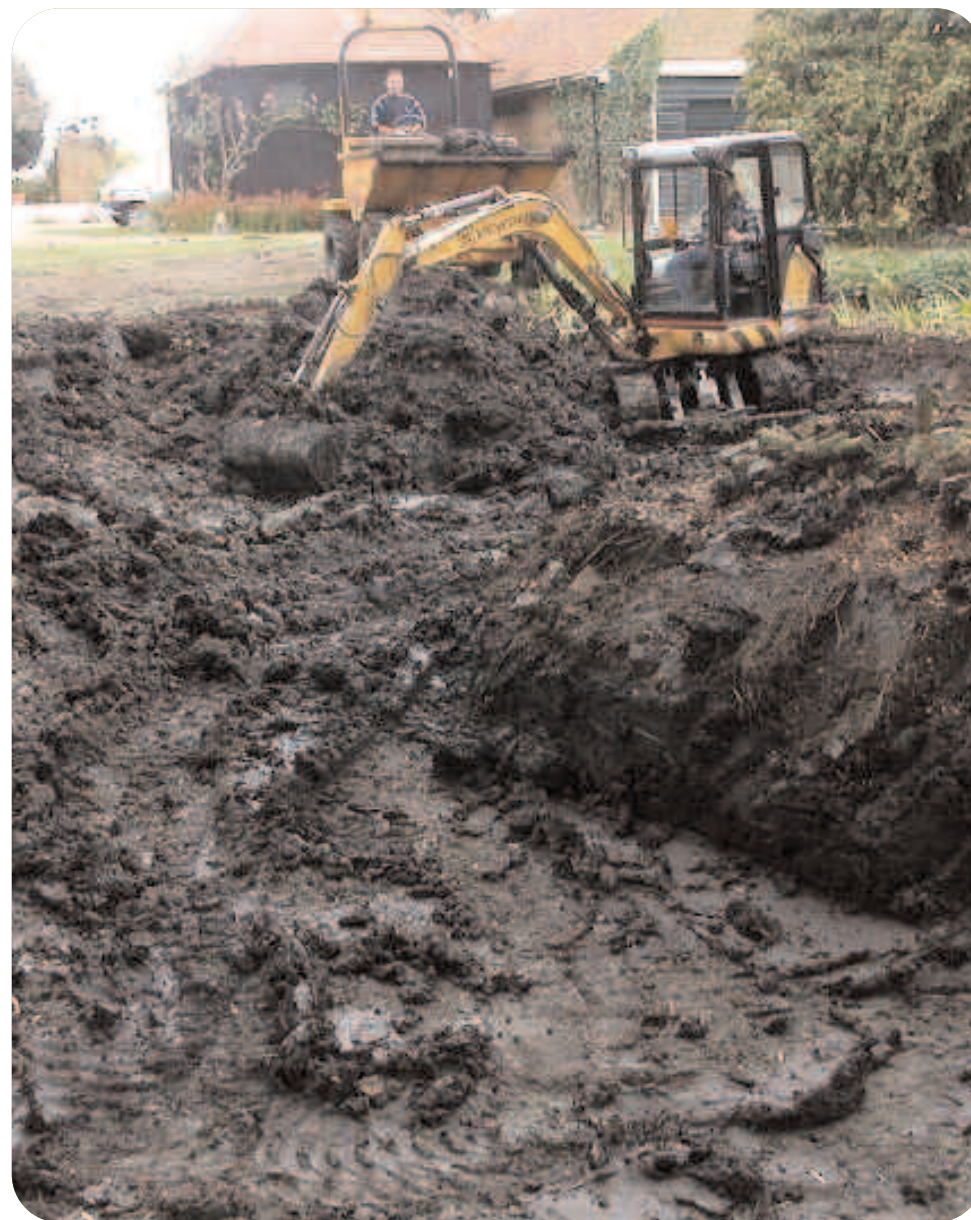
Digging pond by machine. Depending on the size of your pond, you can dig it by hand or machine.
